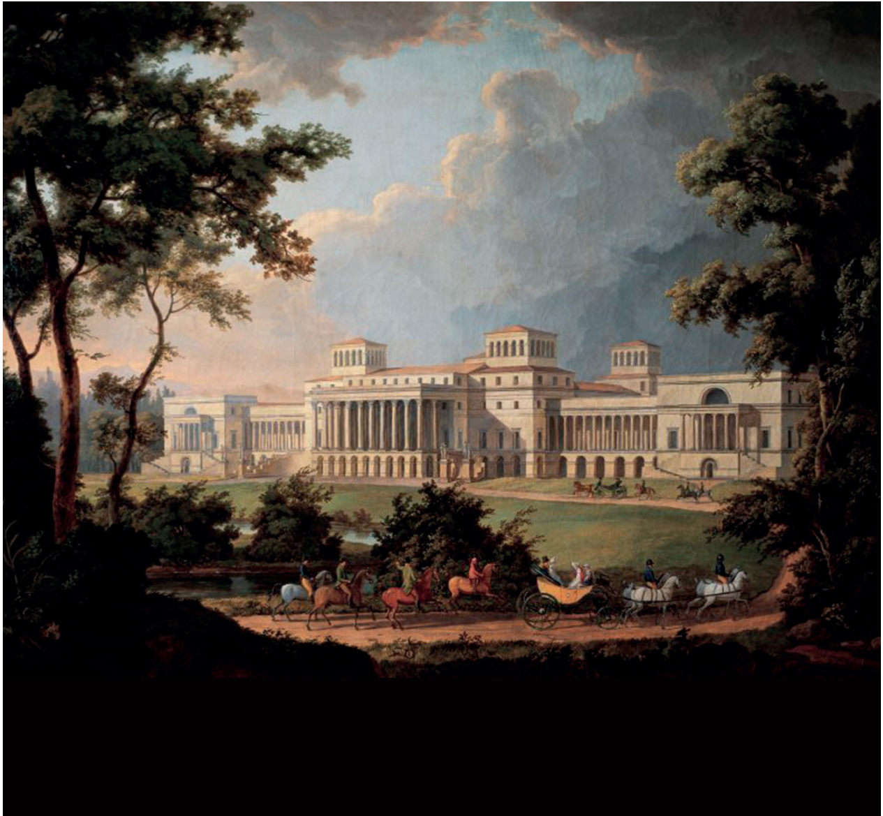
Garden Façade of the Esterházy Palace, Eisenstadt (1812). Painting by Albert Christoph Dies
