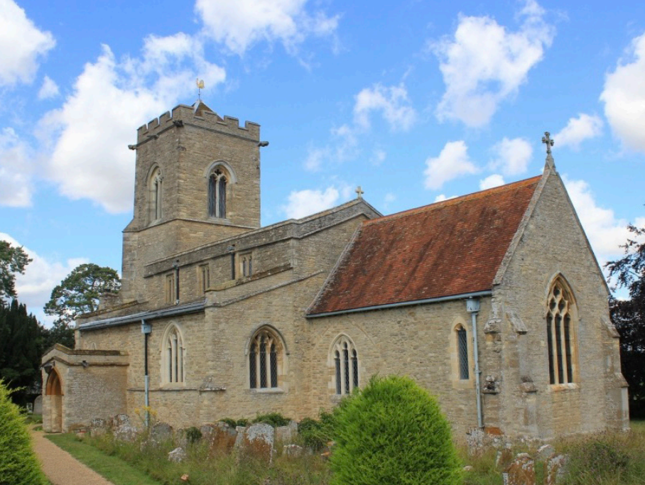
St. Mary's church Carlton, Bedfordshire. England.
